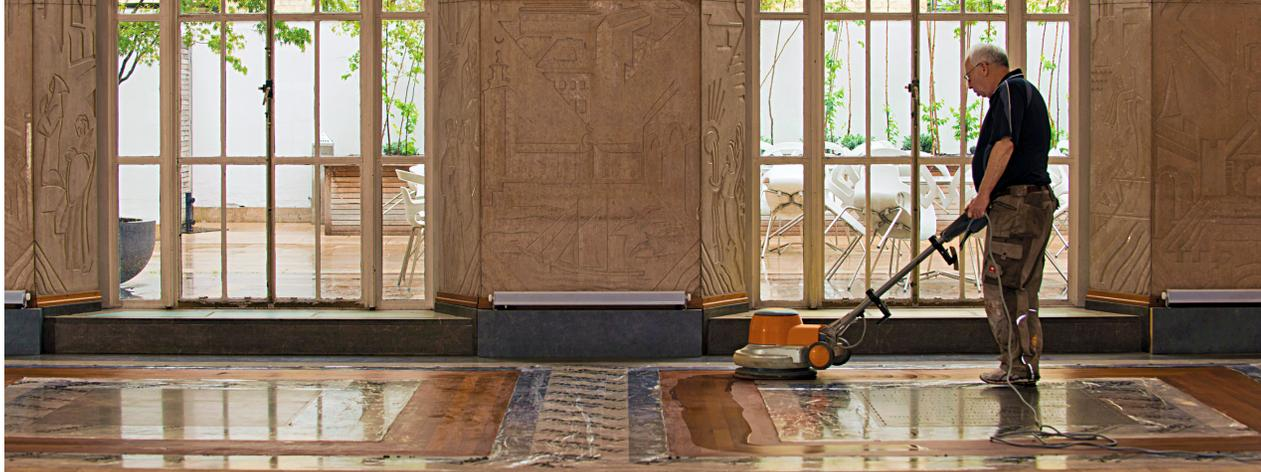
PALLMANN MAGIC OIL 2K ERGO is designed to be a one coat domestic ... two coat commercial system with a longer 40 minutes working time, upright squeegee application.
